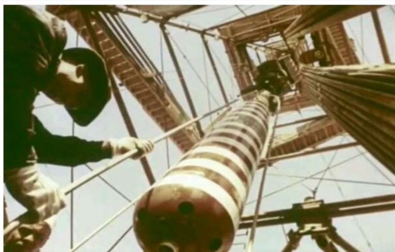
Video image showing USSR nuclear device being lowered into well for detonation shockwave to extinguish runaway oilfield fire. A Russian newspaper reported nuclear blasts first used in 1966 to put out a natural gas well fire in Uzbekistan.
