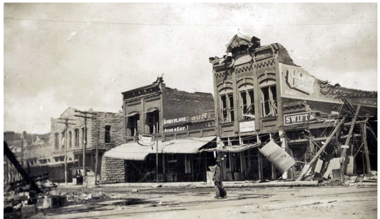
Ardmore Gas Explosion
