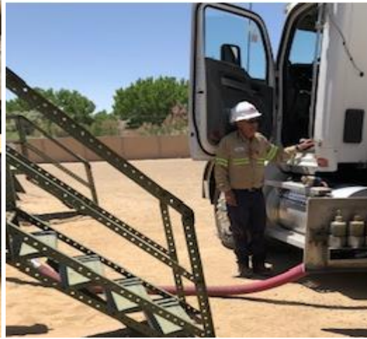
Pump operations, and safety features
