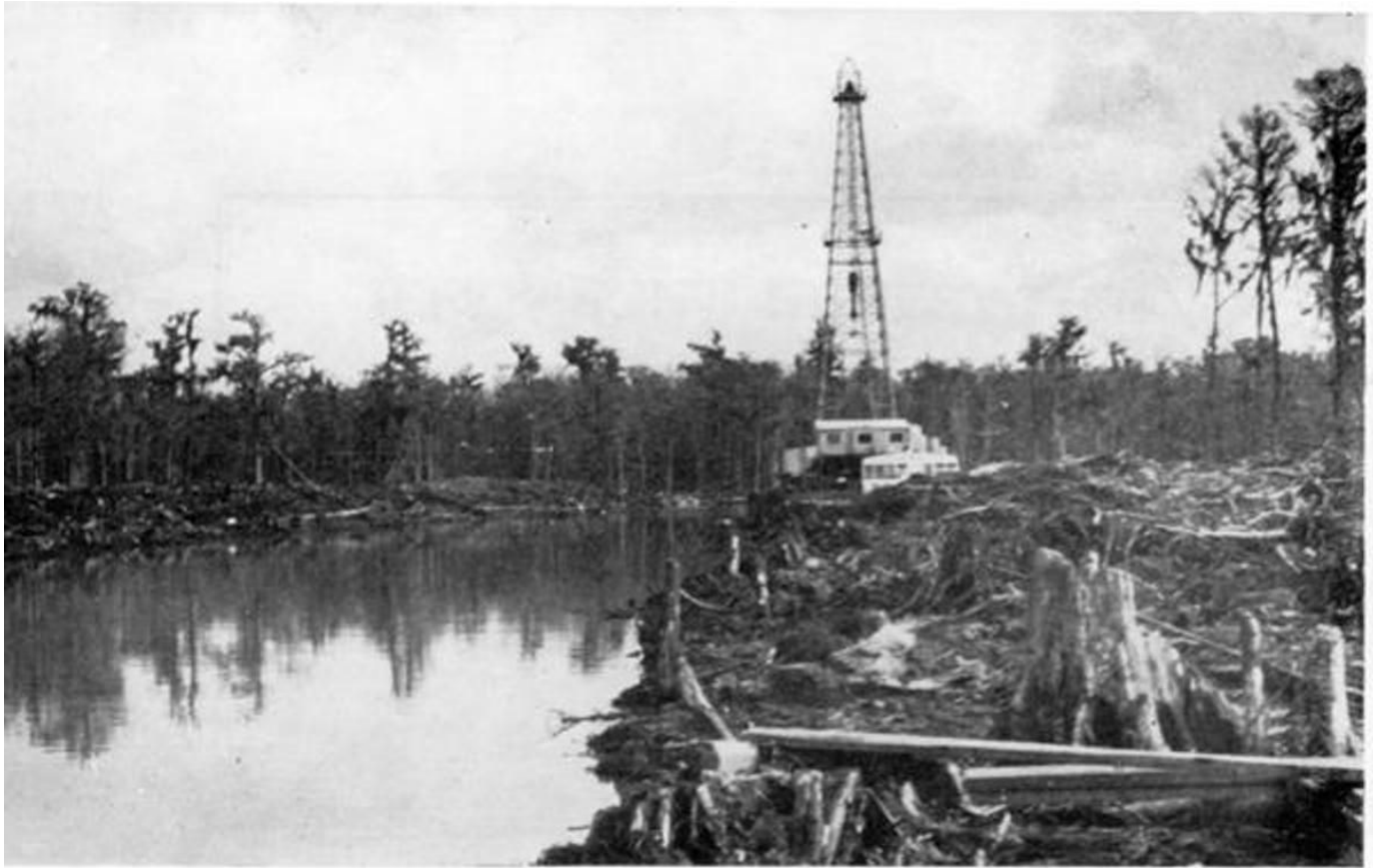
The California Co. drills from barges in the Barataria field. This canal was dug especially to give access to the proposed drill site, as water transport is more feasible than land travel through the marshes. The rig is on a barge, sunk in the canal to give a solid foundation for drilling operations.
